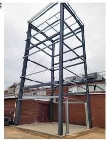
installation area, took soil samples and had an architect, structural engineering, permit expediter, and a construction contractor for the building. Time was spent helping engineers and architects get it right before they completed the design. A 45-foot tall Butler industrial metal structure was used to streamline construction, save time, and a substantial amount of money compared to a conventional block building.
